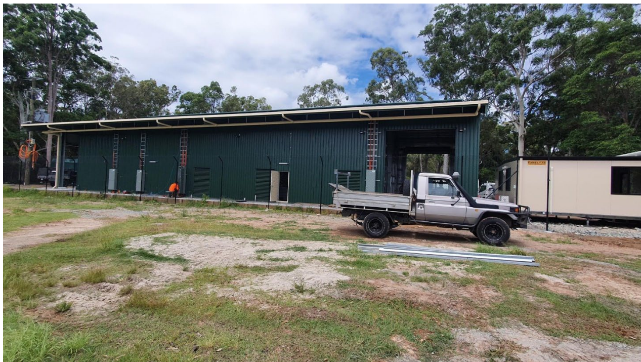
The 440 sq mt, 6 mt high structure is insulated and has passive solar design features to reduce heat load in summer. Set in a greenfields area of the Redlands Research Park workers have sighted koalas in the forest immediately around the site.
