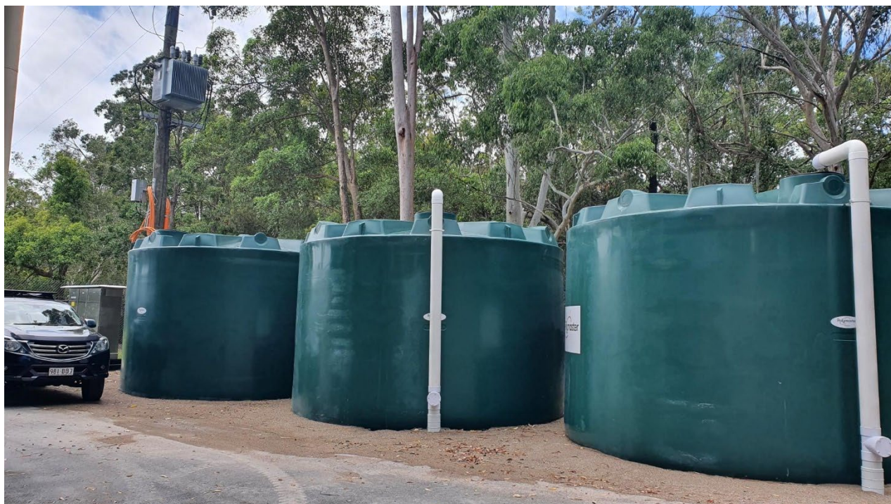
The tank farm both helps manage the significant water catchment of the >500sq mt roof as well as provide rain water for use in process and cooling water.
