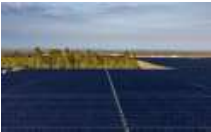
50MW Kidston Solar
